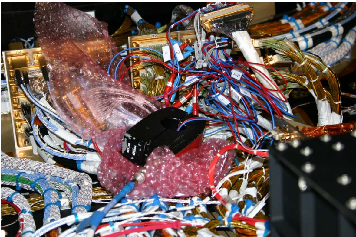
picture 2 CM Current measurement FD on power lines
