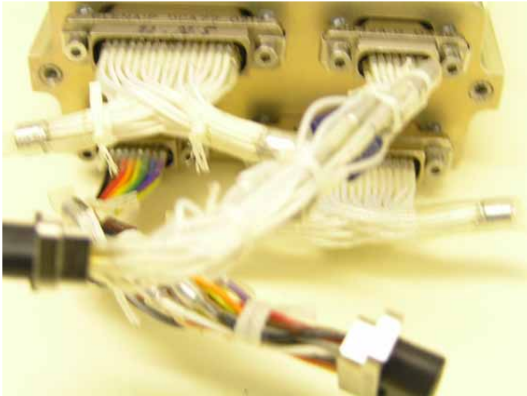
Rear view showing Tails & terminators in place
