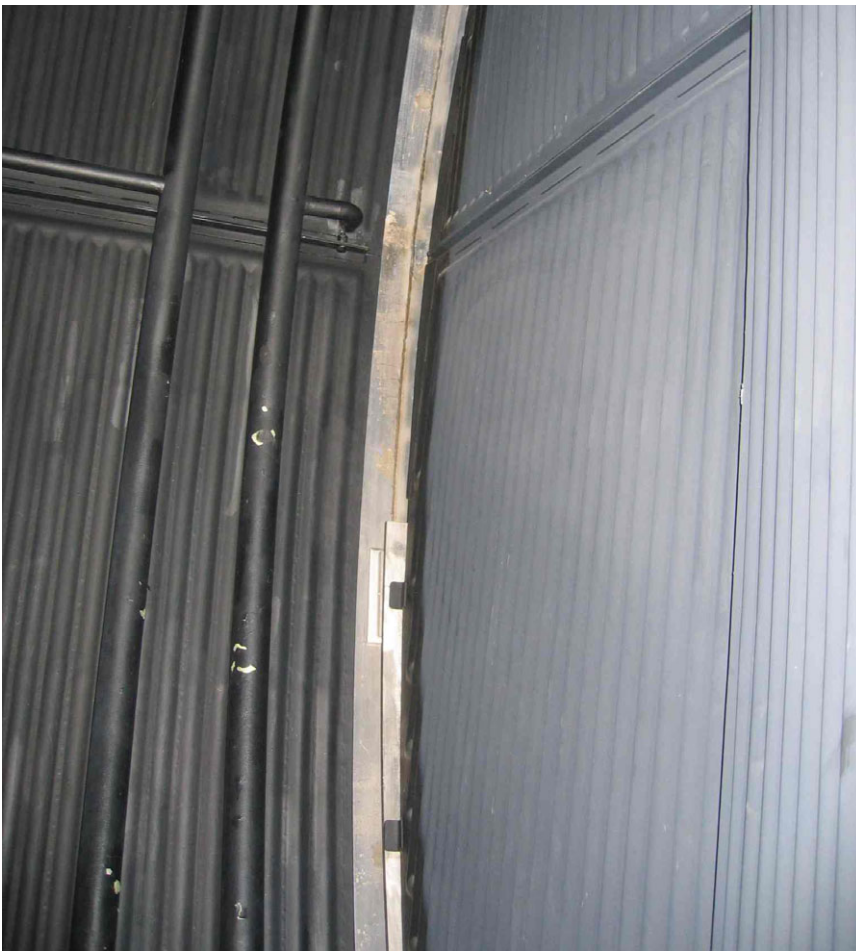
Figure 6.4-10: Circumferential gap around 5m door shroud
