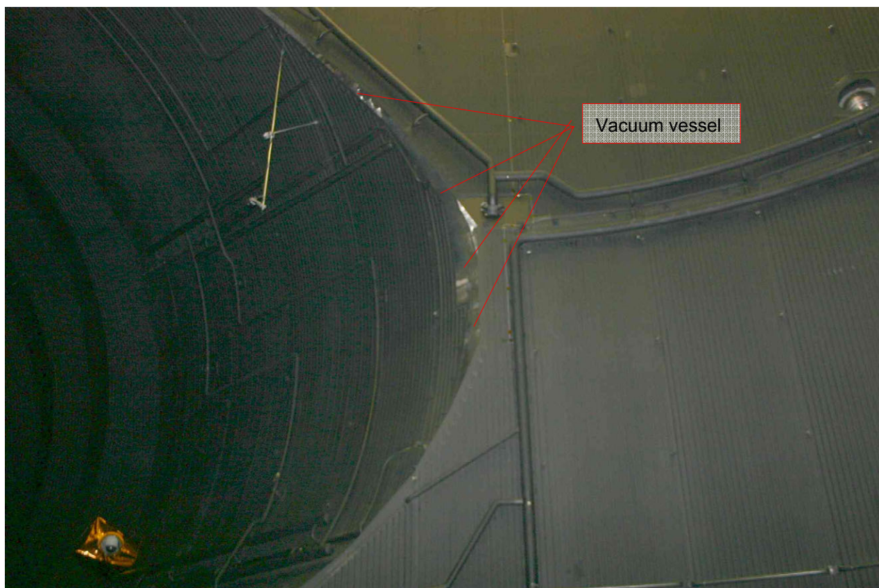
Figure 6.4-4: Shroud gaps in nozzle connection to cylinder
