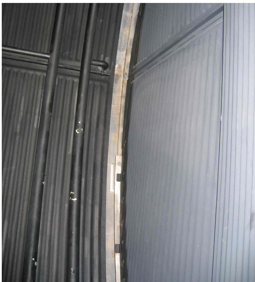
Figure 6.4-10: Circumferential gap around 5m door shroud
