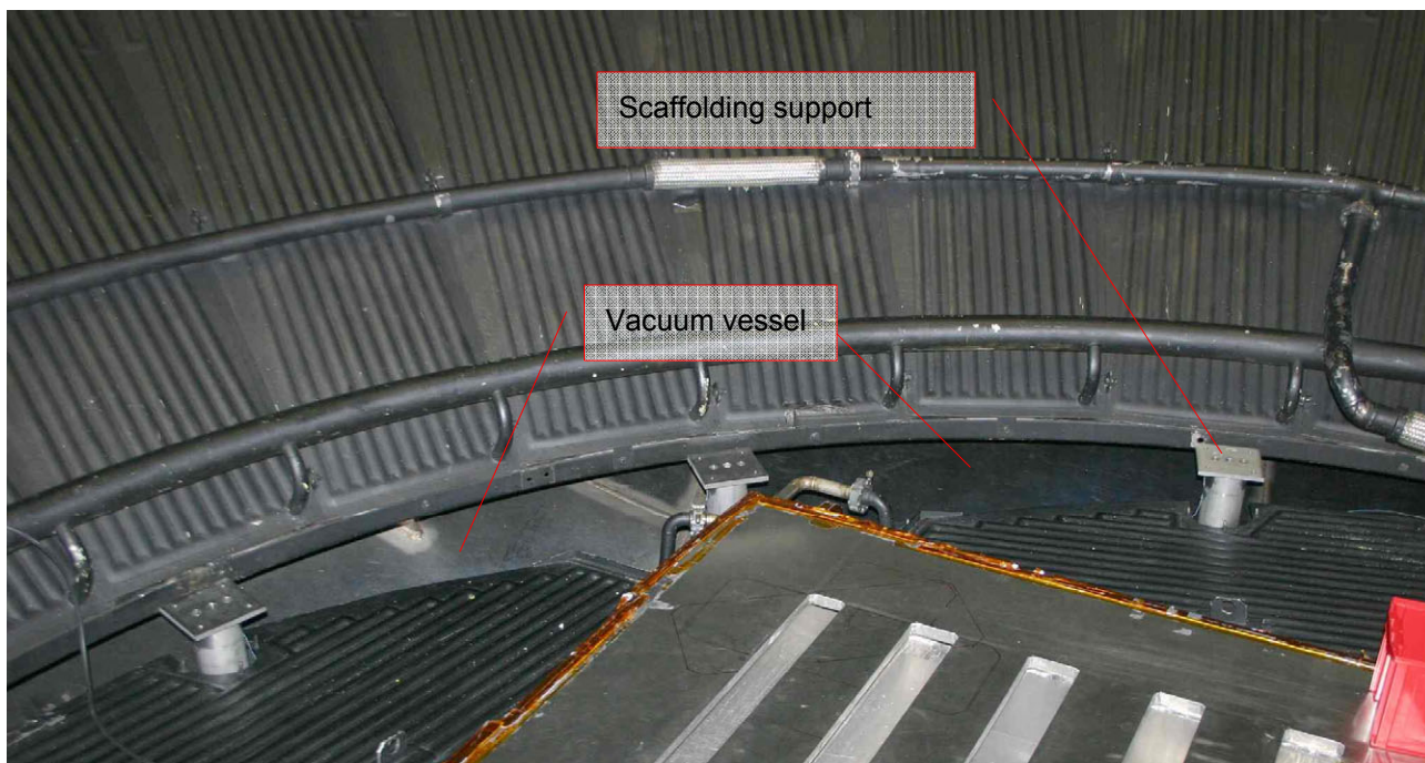
Figure 6.4-3: Scaffolding supports and view to vacuum vessel
