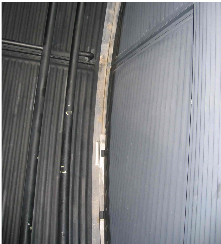
Figure 6.4-10: Circumferential gap around 5m door shroud
