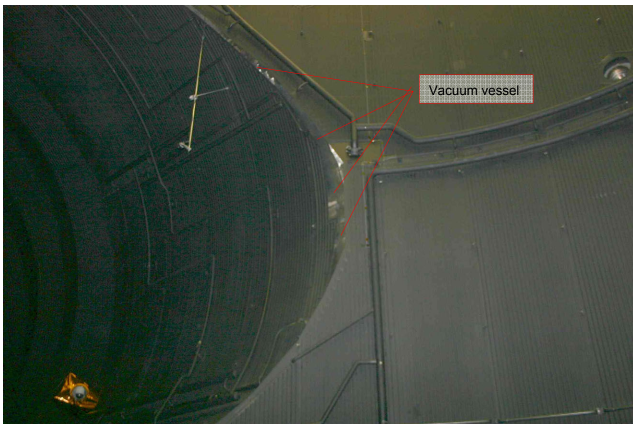
Figure 6.4-4: Shroud gaps in nozzle connection to cylinder
